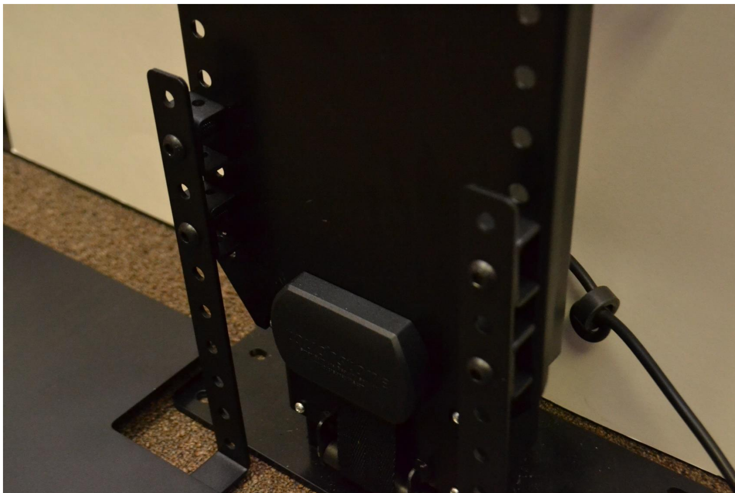
Shelf brackets installed.
